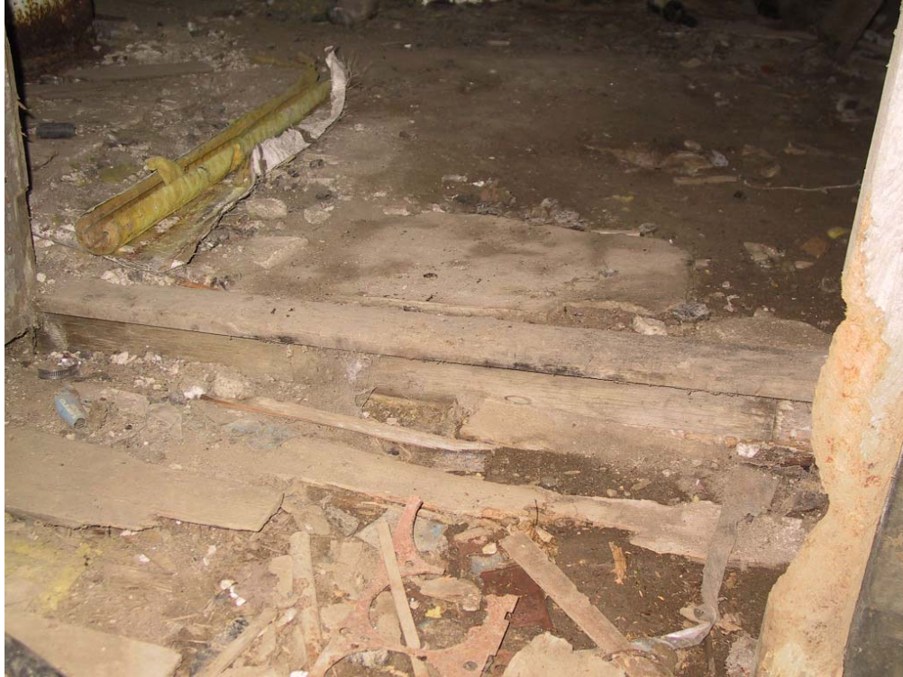
Wood threshold in Room B102 to Room B103. Evidence suggests that there may have been a wood plank floor in Room B102.
