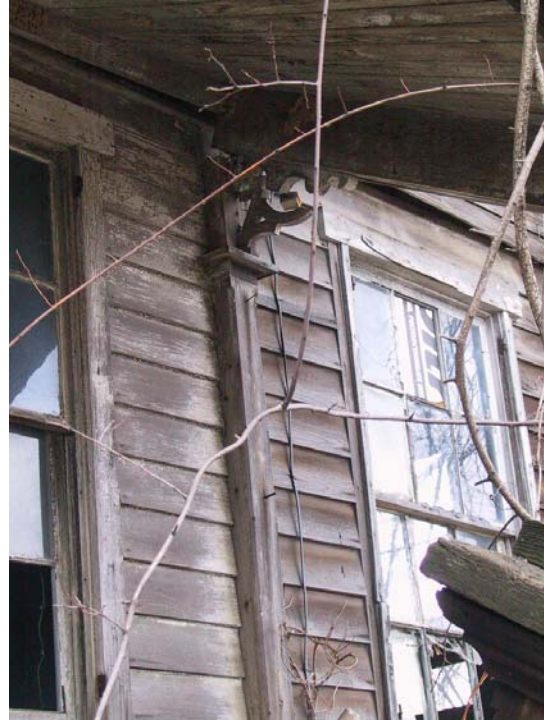
Front porch pilaster and bracket
