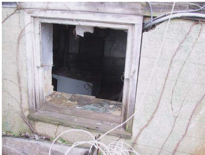
Southeast cellar window surrounded by scored stucco finish over the masonry foundation
