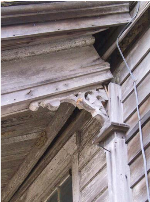
Front porch pilaster and entablature
